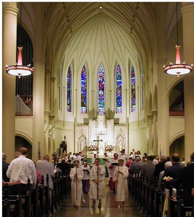
In the interior of St. Mary's Episcopal Cathedral, Hord Architects brought in new mechanicals, supplemented pendant lights, adjusted pews, designed new modesty rails and restored plasterwork. Photo: courtesy of Hord Architects
