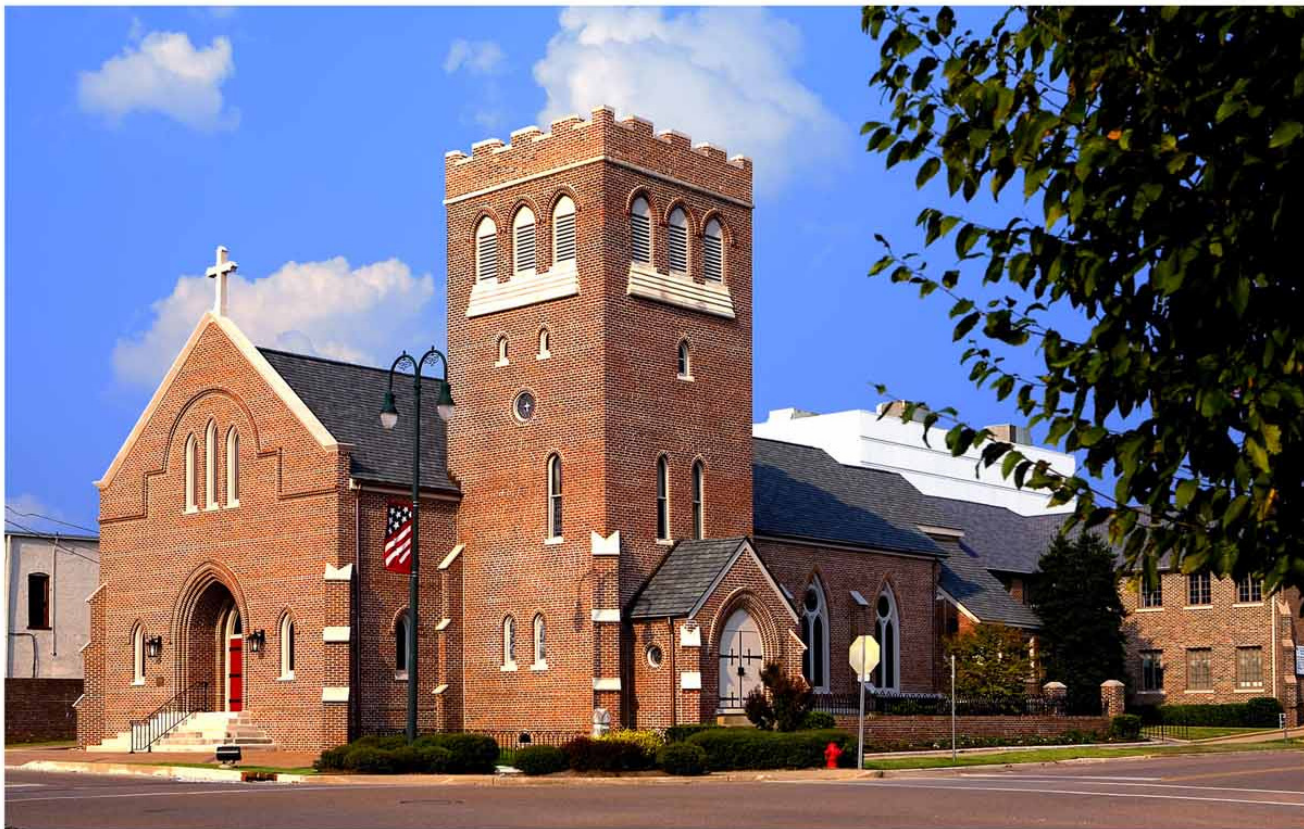
St. Luke's Episcopal Church in Jackson, TN, an 1840s landmark, reopened this fall, after Hord Architects undid devastating 2003 tornado damage. Photo: ©2006 Jeffrey Jacobs Photography
